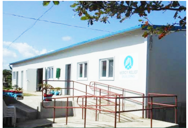
Mercy Relief building in SHS Palo, Leyte, turned over January 2016
