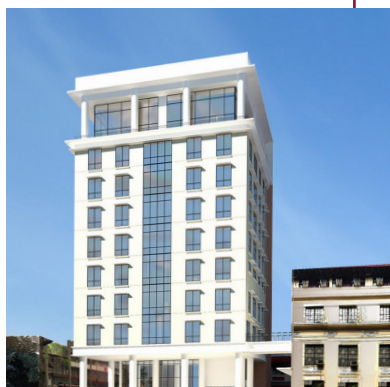
CPH Dr. Stephen Zuellig Hall project implementation has been put on hold with the demise of the donor
